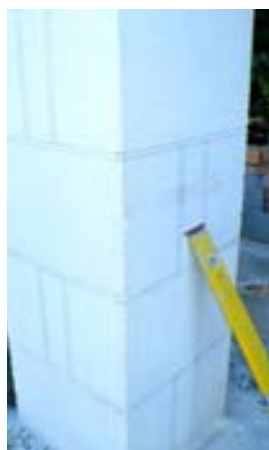
Traçage des joints
